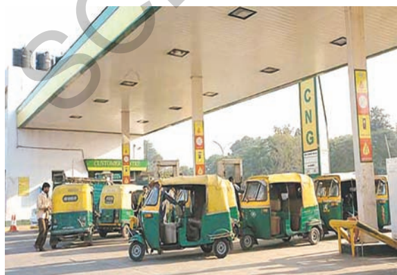
Fig - 3: CNG filling station
